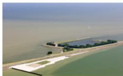
Houtrib Dike Pilot Project
