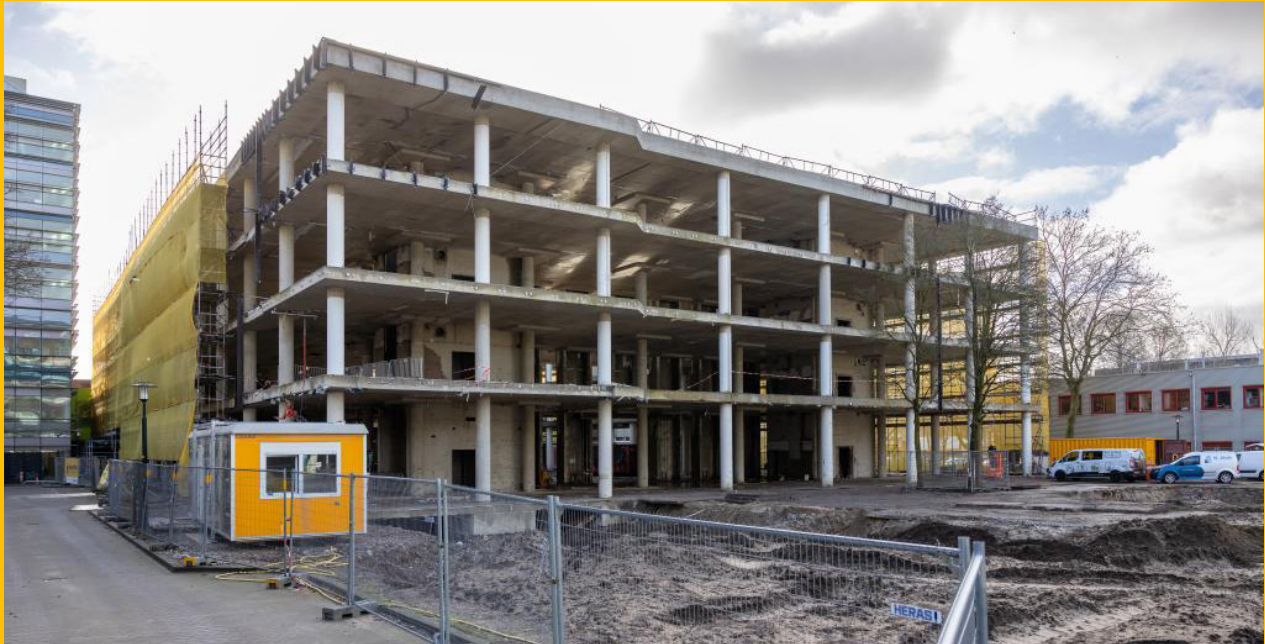
Photo: demolition earth sciences building
