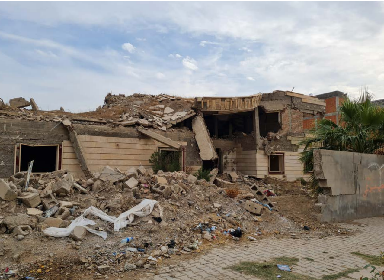
Figure 8: Damaged houses next to the industrial neighbourhood, November 2021. PAX/Saba Azeem.
