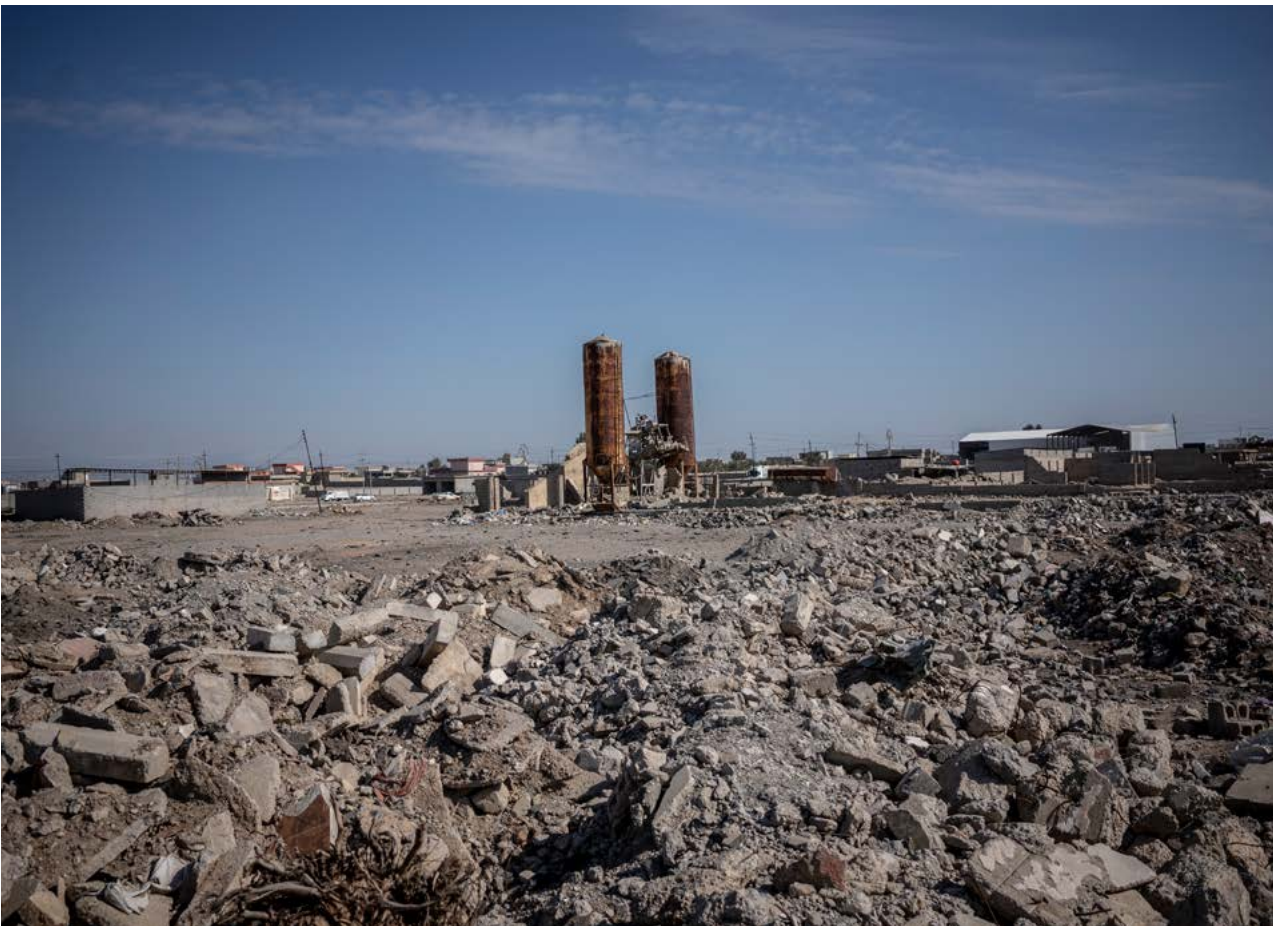
Figure 10: The brick factory which got damaged in the June 2015 airstrike, February 2022. PAX/Ayman al-Amiri.
